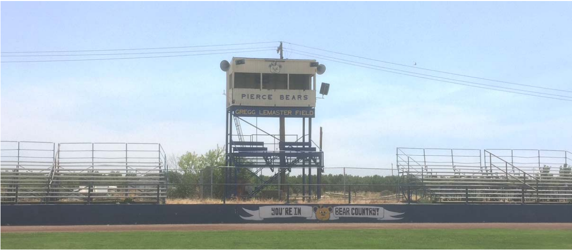
Existing Bleacher System
